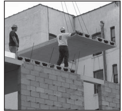
Putting a steel-reinforced concrete plank in place
