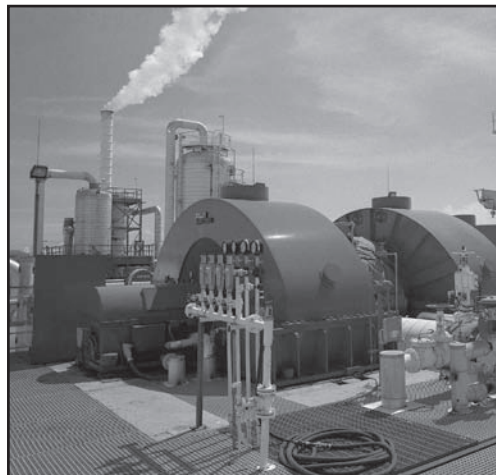
The Leathers Geothermal Power Plant in Calipatria, CA
